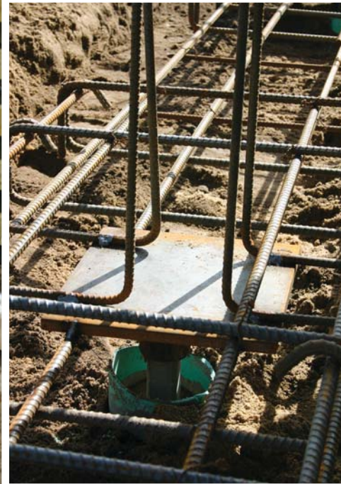
Figure 4. Bearing plates (above) are welded to the top of each shaft, just above grade. Vertical rebar dowels, welded to the bearing plates, provide continuity from the pier through the grade beam and stem-wall foundation.
