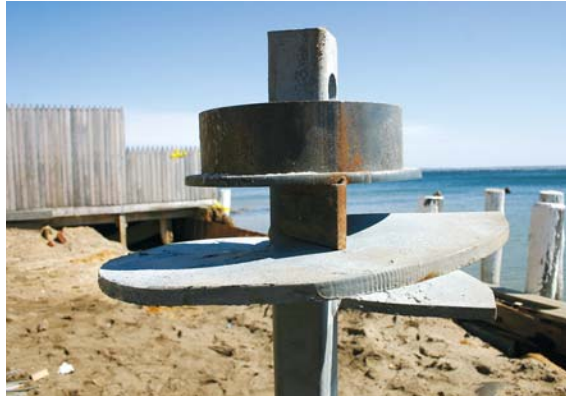
Figure 2. Helical piers don't remove material the way an auger does; instead they screw into the soil with minimal disturbance. A displacement plate, shown here upside down (top left) and added to the top of the lead section (top right), creates a void around the shaft as it is screwed into the ground. A 6-inch-diameter PVC casing fits onto the displacement plate and is pressed into the soil along with the first plain shaft section (bottom left). Incremental marks on the casing allow the insertion torque to be tracked at 1-foot intervals. Grout is poured in as each additional section is coupled and driven (bottom right).
