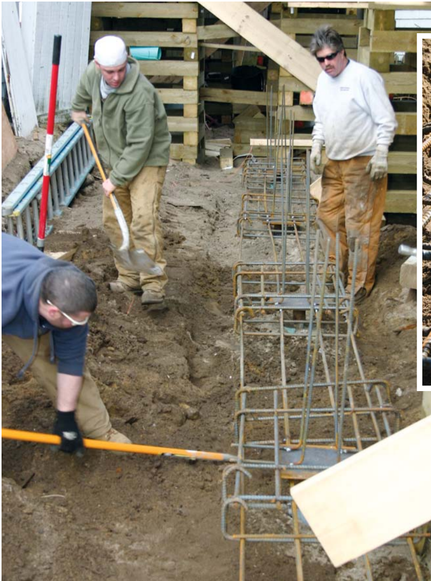
Figure 4. Bearing plates (above) are welded to the top of each shaft, just above grade. Vertical rebar dowels, welded to the bearing plates, provide continuity from the pier through the grade beam and stem-wall foundation.
