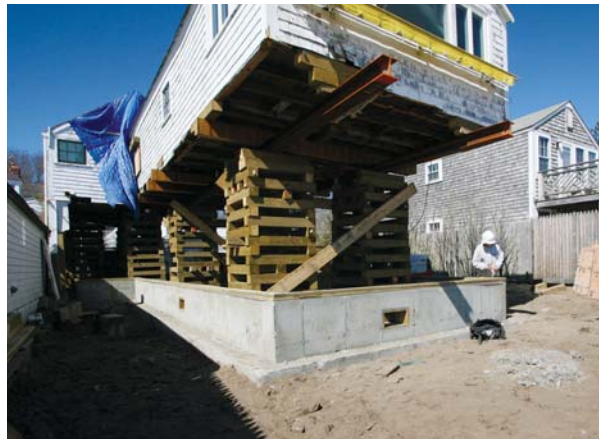
Figure 5. The excavator operator guides concrete placement for the stem wall (top), which is tied to the grade beam with a hefty schedule of vertical rebar (above). Note the knockouts for the required storm vents (right).
