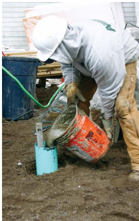
Figure 2. Helical piers don't remove material the way an auger does; instead they screw into the soil with minimal disturbance. A displacement plate, shown here upside down (top left) and added to the top of the lead section (top right), creates a void around the shaft as it is screwed into the ground. A 6-inch-diameter PVC casing fits onto the displacement plate and is pressed into the soil along with the first plain shaft section (bottom left). Incremental marks on the casing allow the insertion torque to be tracked at 1-foot intervals. Grout is poured in as each additional section is coupled and driven (bottom right).
